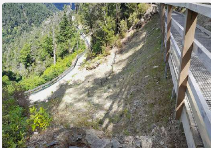
(Below) the Dunn slip face had over $5,000 of natives planted on it, but after 2-3 years regrowth is minimal due to high pressure from grazing animals such as goats, deer and possum. The native plantings have little chance of survival if pests are not controlled.
