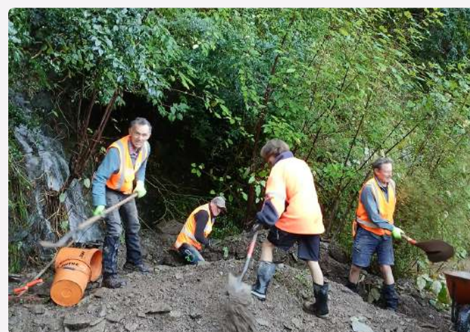
Digging out a culvert to keep the storm water flowing
