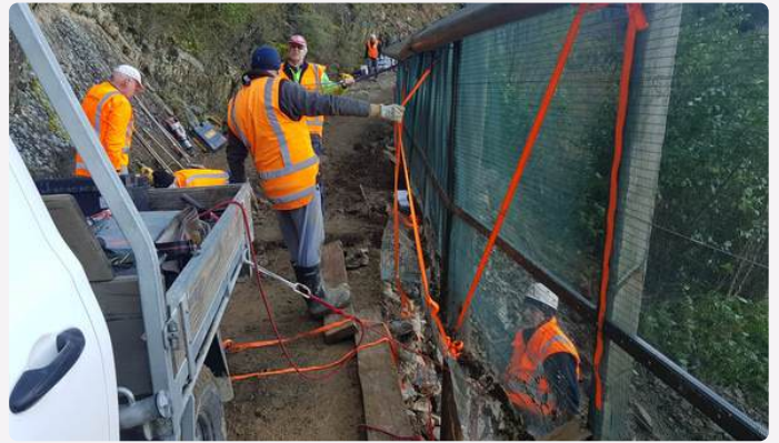
Fence and assets team strengthening the damaged fence
