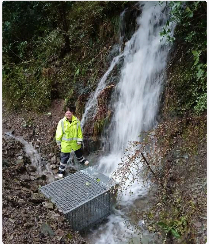
Chelsea standing next to new culvert with opening front
